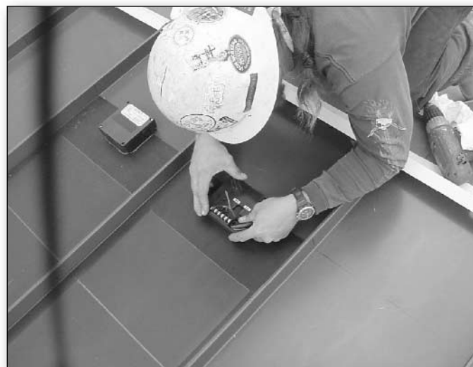
Locating and installing the PVL junction box
