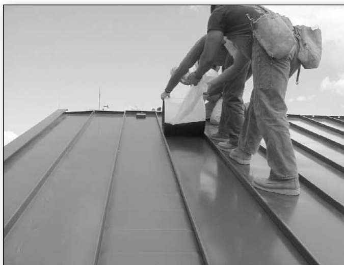
Removing the backing and unrolling Uni-Solar PVL solar panels
